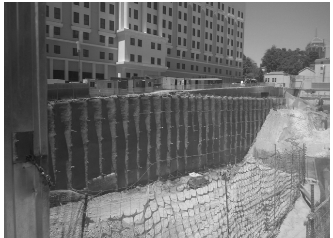
Figure 1. Multi-anchored soldier pile wall at The Marc
